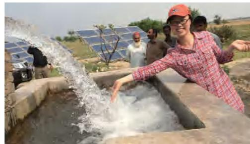
System: 37kw solar pump system
