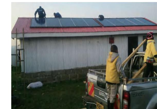
System Solution: 2.2kw Solar Pump System
