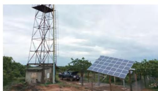
System: 3.7kw solar pump system
